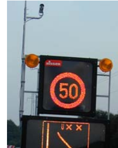
Figure 14: A temporary mobile incident detection system on a French highway
